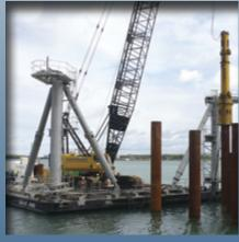
Driving piles into a seabed requires great accuracy in a harsh environment. Trimble Site Positioning Systems utilize precision GNSS, heading sensors, and integrated software to get the inh done right
